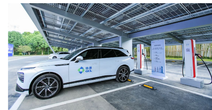
The "photovoltaic+storage+charging" energy station in the GCL Energy Center provides employees with "one second, one kilometer" supercharging
