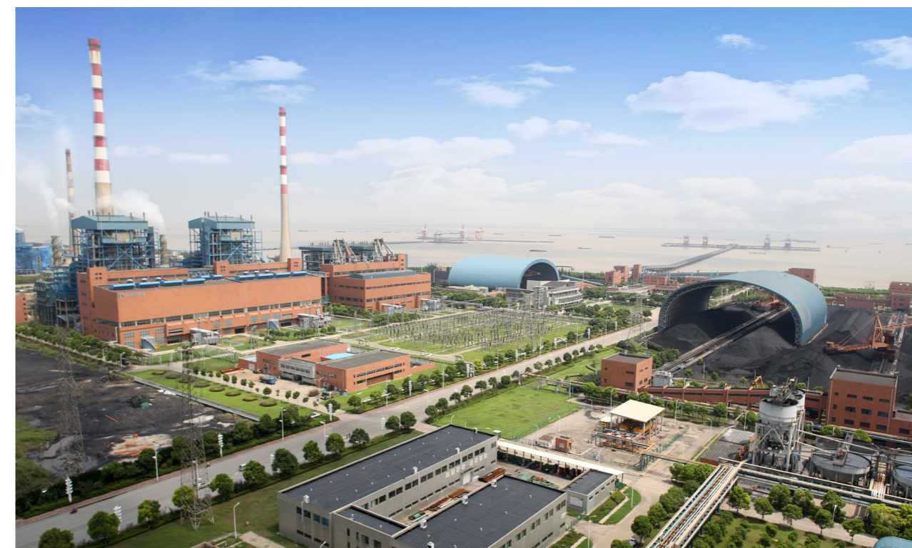
Interior of Taicang Port Power Plant
