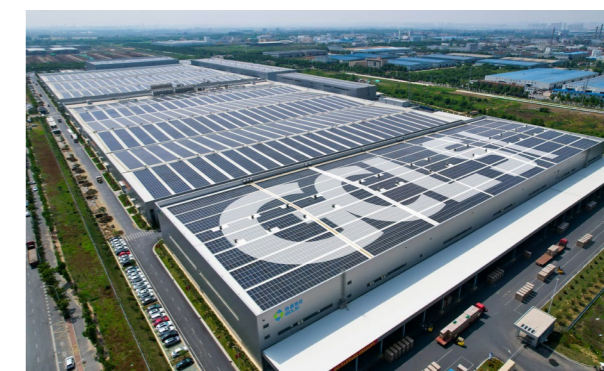
Hefei GCL Xinyu Photovoltaic Power Station
